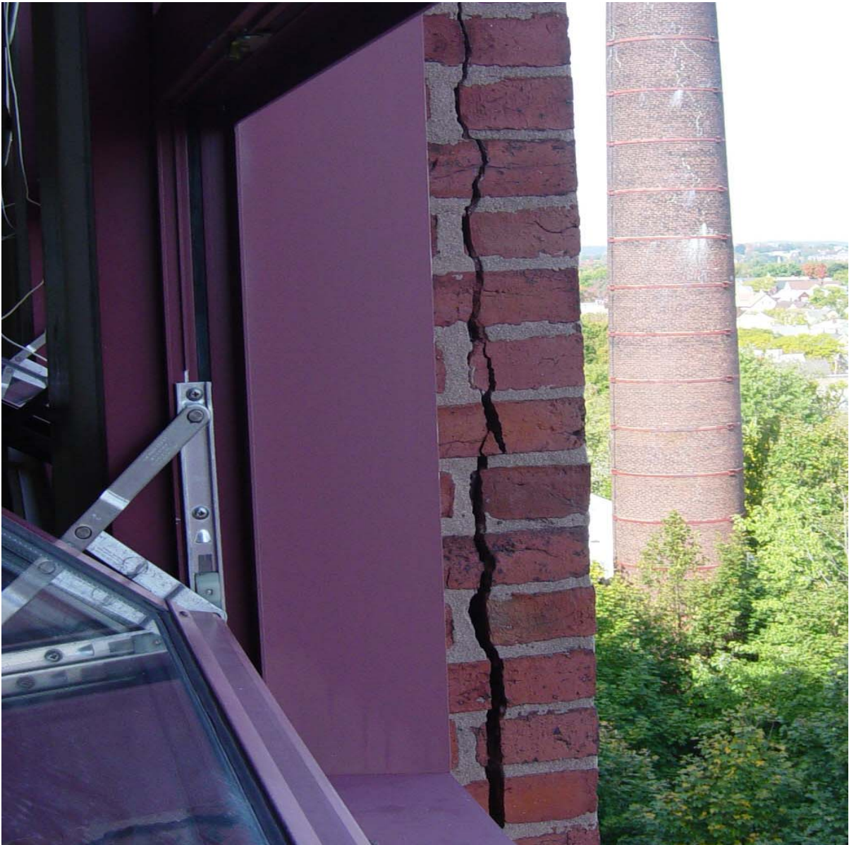
Exterior face of brick is breaking away at pier between windows, a common occurrence
