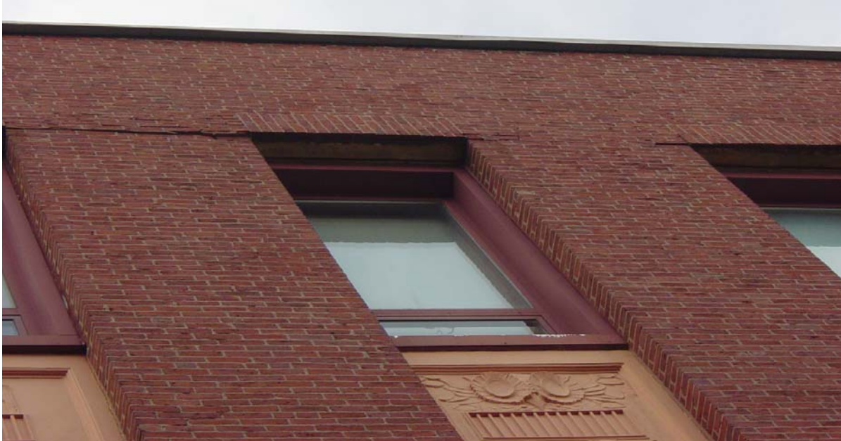
Photo 25 - Rear of building. Face brick is moving outward above windows, causing cracking as seen. At several locations, brick has moved to the edge of the lintel at the window head. Eventually this could lead to the brick falling off. We recommend removal and rebuilding of the effected wall areas.
