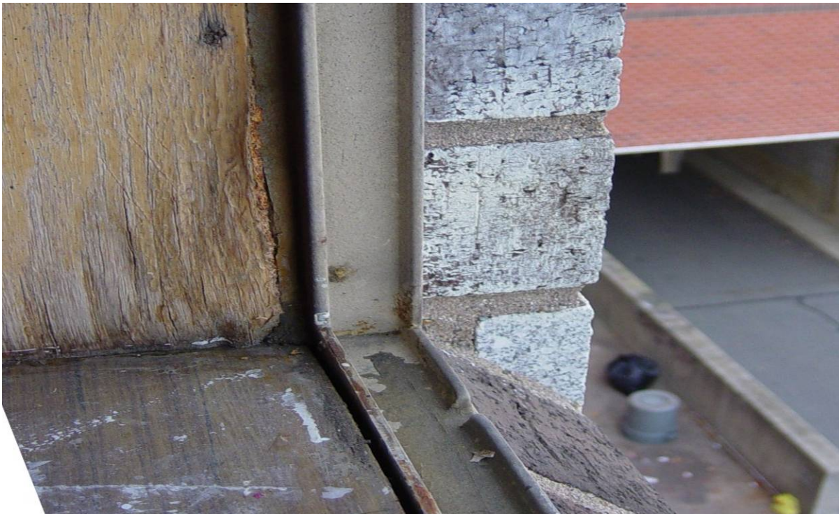
Photo 38 - Painting and Decorating Shop. Some windows show severe deterioration at the jambs due to moisture; others do not. Indicates improperly sealed air/vapor barrier.
