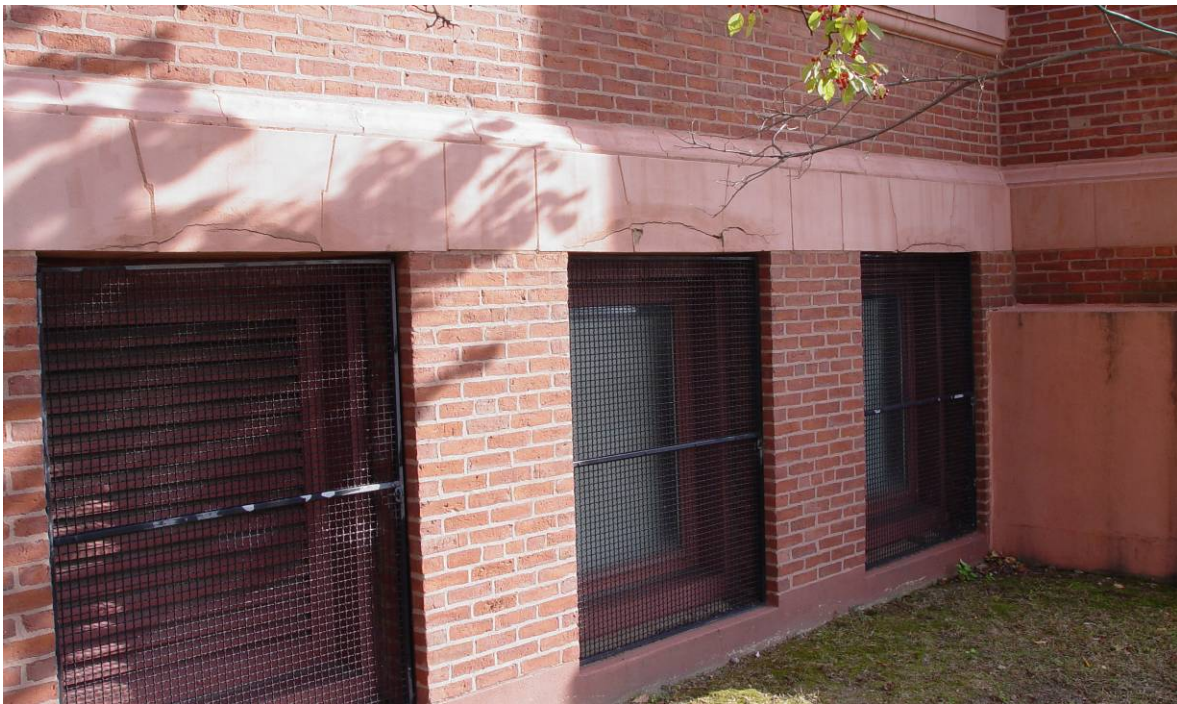
Photo 2 - Cracking of stone lintels, previously repaired, typical at approximately 12 windows.
