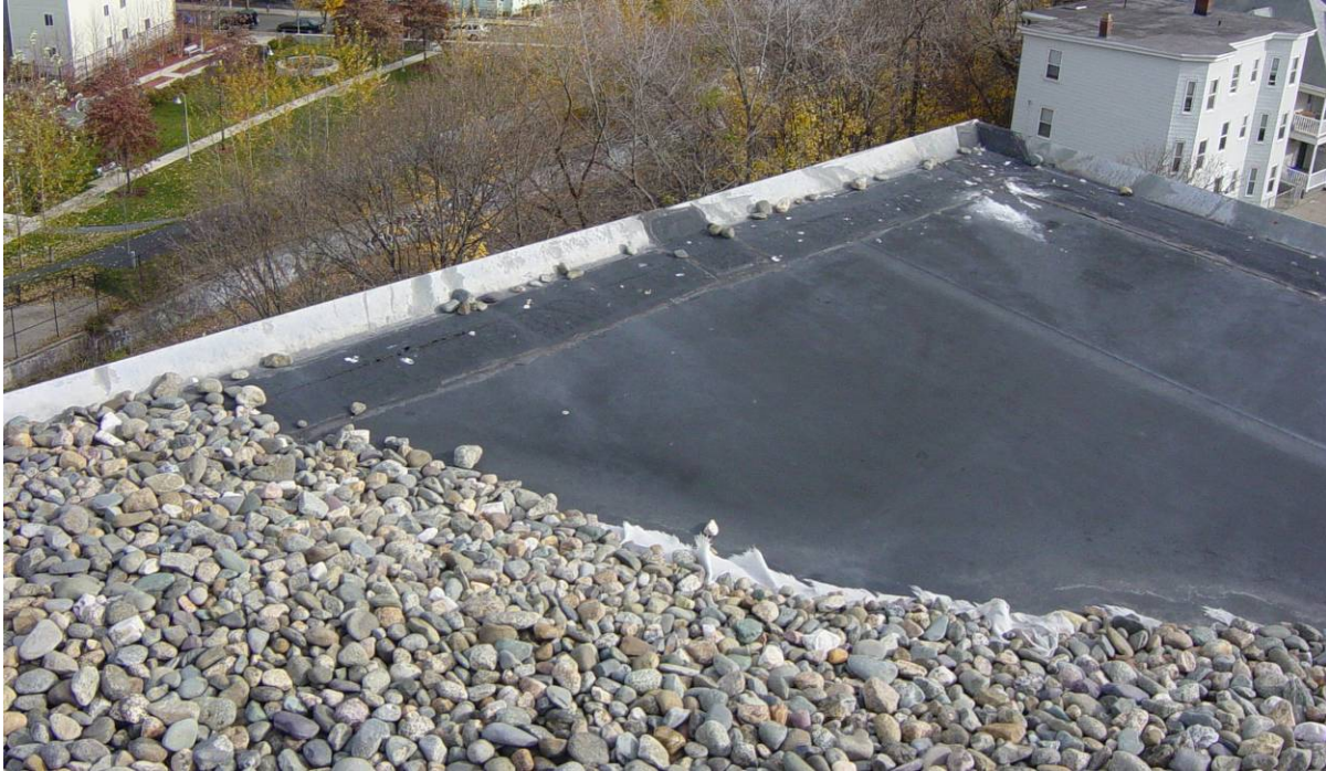
Photo 49 - Gymnasium. Wind has dislocated ballast and torn the protection fabric at the northeast and northwest corners. EPDM membrane is cracked and deteriorated along the perimeter edge, but appears to be in good condition where covered.
