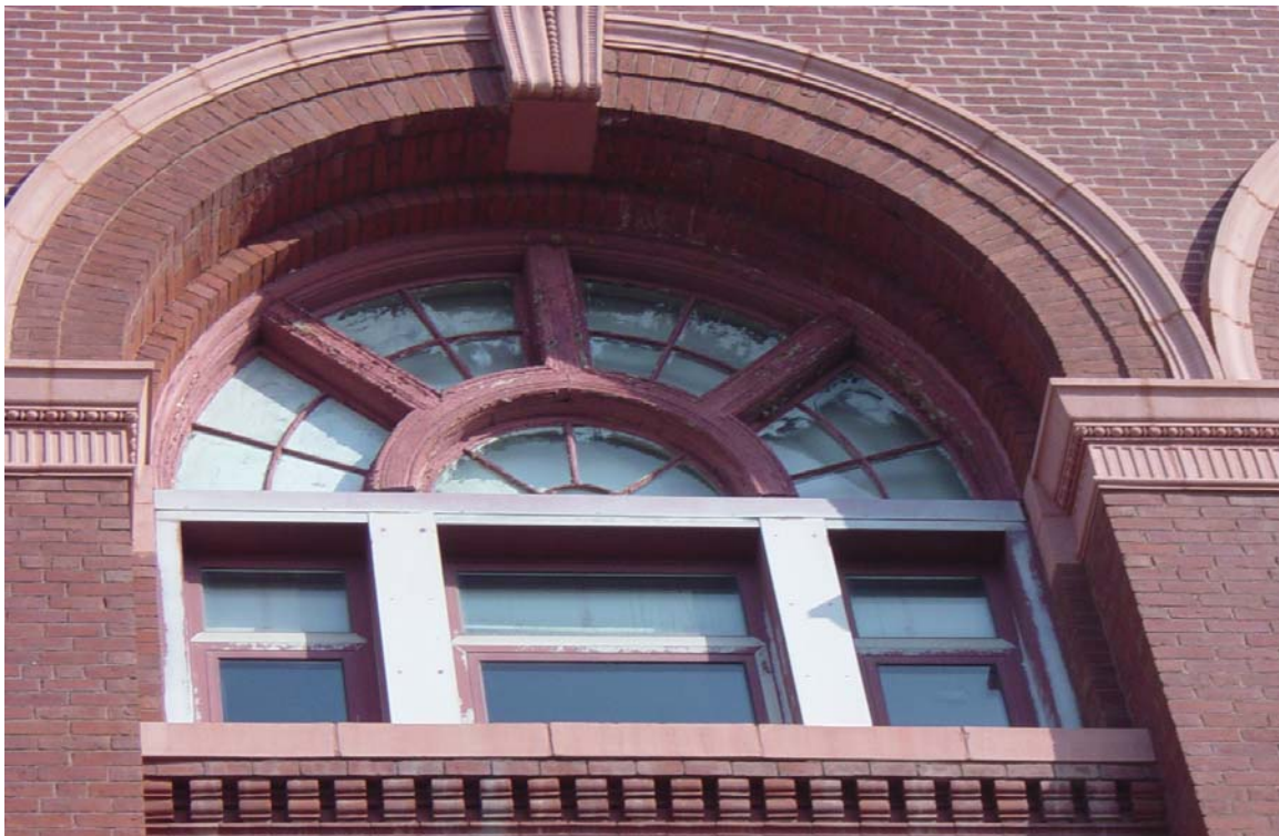
Current photo, showing deterioration and poor aesthetic match of windows installed in 1986
