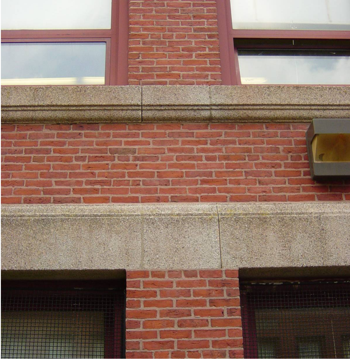
Photo 27 - Rear of building. Previous repointing job appears to have held up well in some areas, but is very soft. Sand easily rubs off the surface of the mortar. Joints were not compacted or tooled. The joints are quite absorptive and allow for easy ingress of water into the wall.
