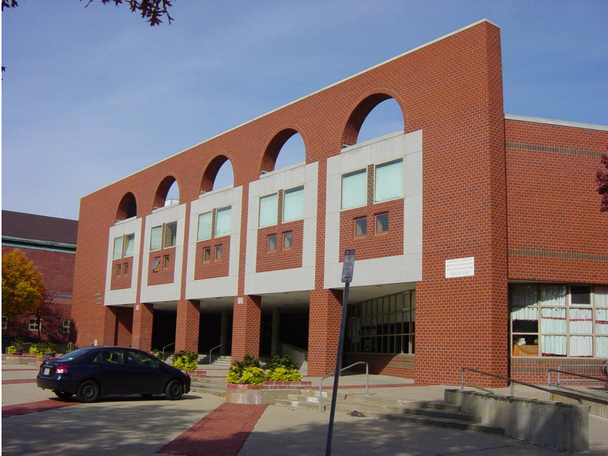
Photo 33 - Technical High School entrance. Cracked and spalled areas of plaza concrete and brickwork need repair or replacement. Sealant joints at slabs have failed and need to be replaced. Some handrails are missing at some steps, and need to be provided. Existing galvanized steel rails are beginning to rust. Brick planters are crudely constructed and poorly detailed, causing damage to the concrete, and need to be replaced.
