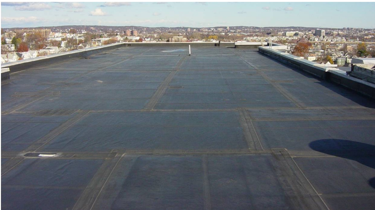
Photo 42 - Central wing, northwest (northeast is similar). Some areas of roof have been “stripped in”, adding EPDM flashing on top of all joints, in an effort to reduce leaks and extend the service life of the roof. Adhesive bond between the membrane and insulation is failing in some areas.
