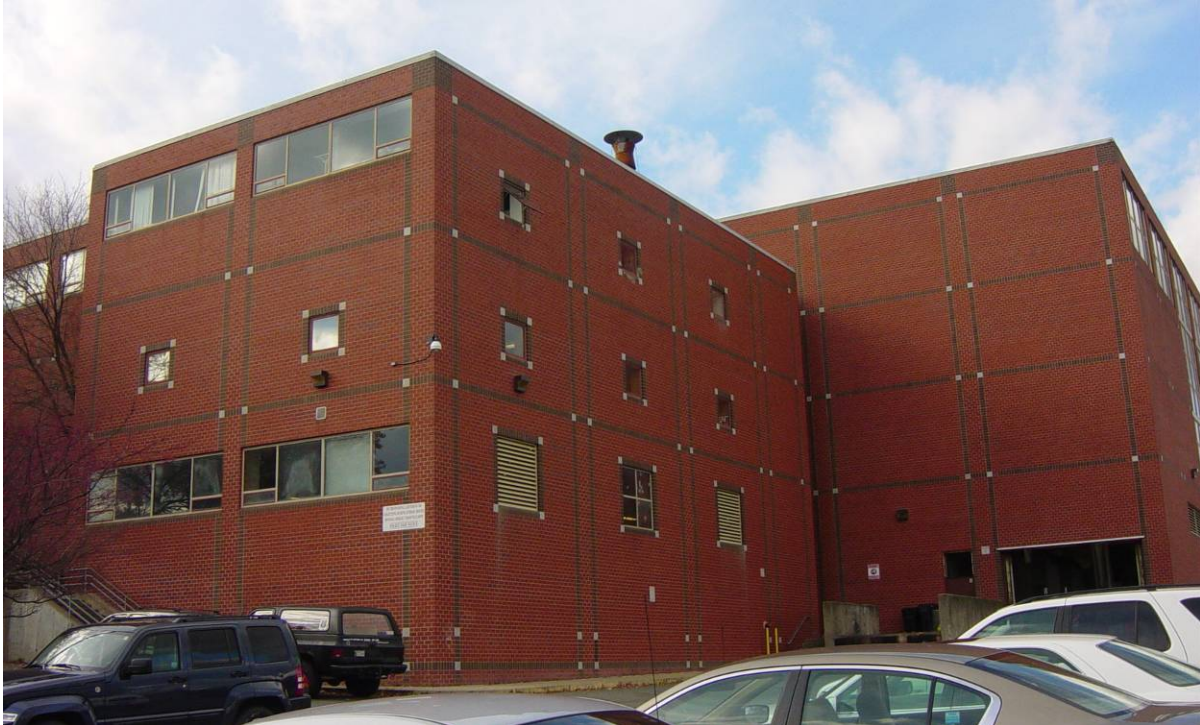
Photo 35 - Rear of Technical High School. Windows lack head flashing and weeps, causing severe damage to interior wood trim.
