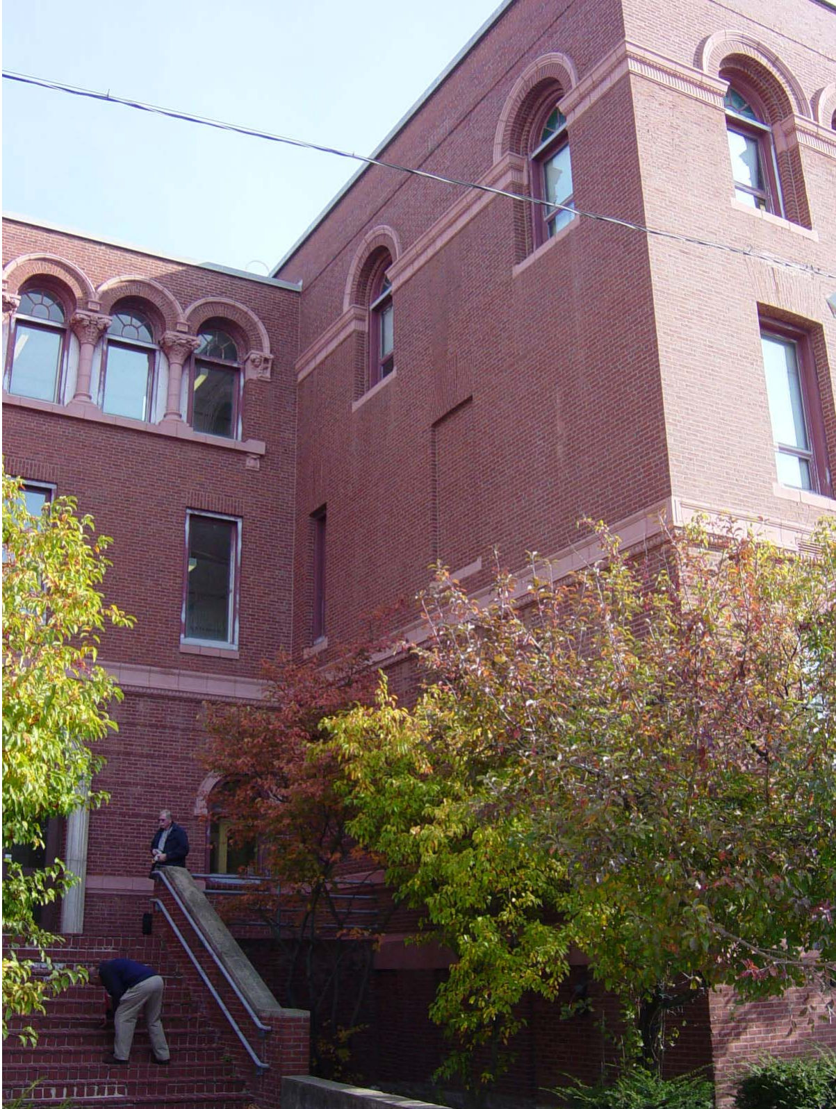
Photo 8 - Wall appears in good condition. Since the initial field investigation, the masonry steps and cheek wall have been repaired.
