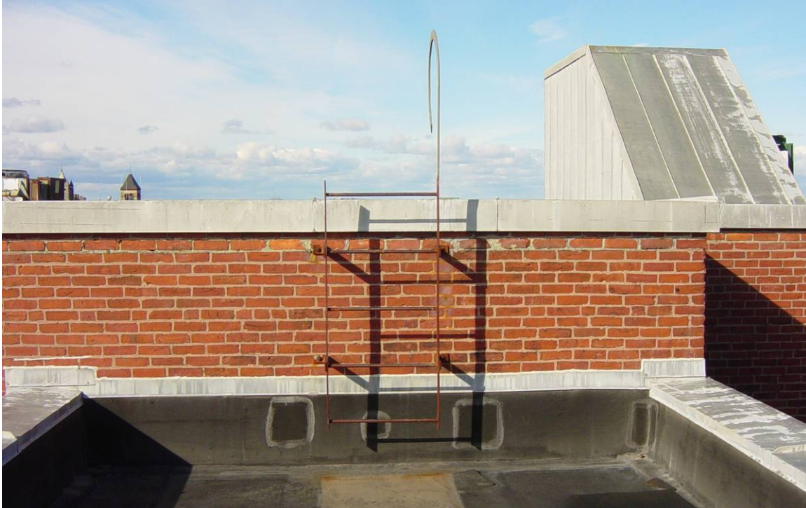
Photo 41 - Link/west entry roof. Like most access ladders at the High School, this one is damaged and not OSHA compliant. Replacement is recommended.
