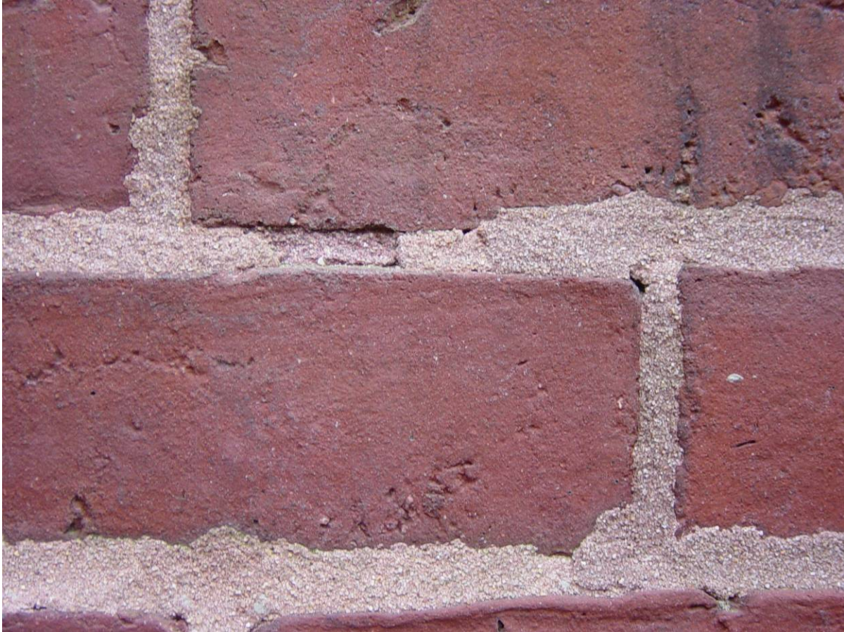
Photo 28 - Rear of building. When the building was previously repointed (date not known), new mortar was applied in a very thin layer (approximately 1/8" thick) over the old mortar. At the center of the picture above, a small area of newer mortar has popped off, revealing the original mortar below.
