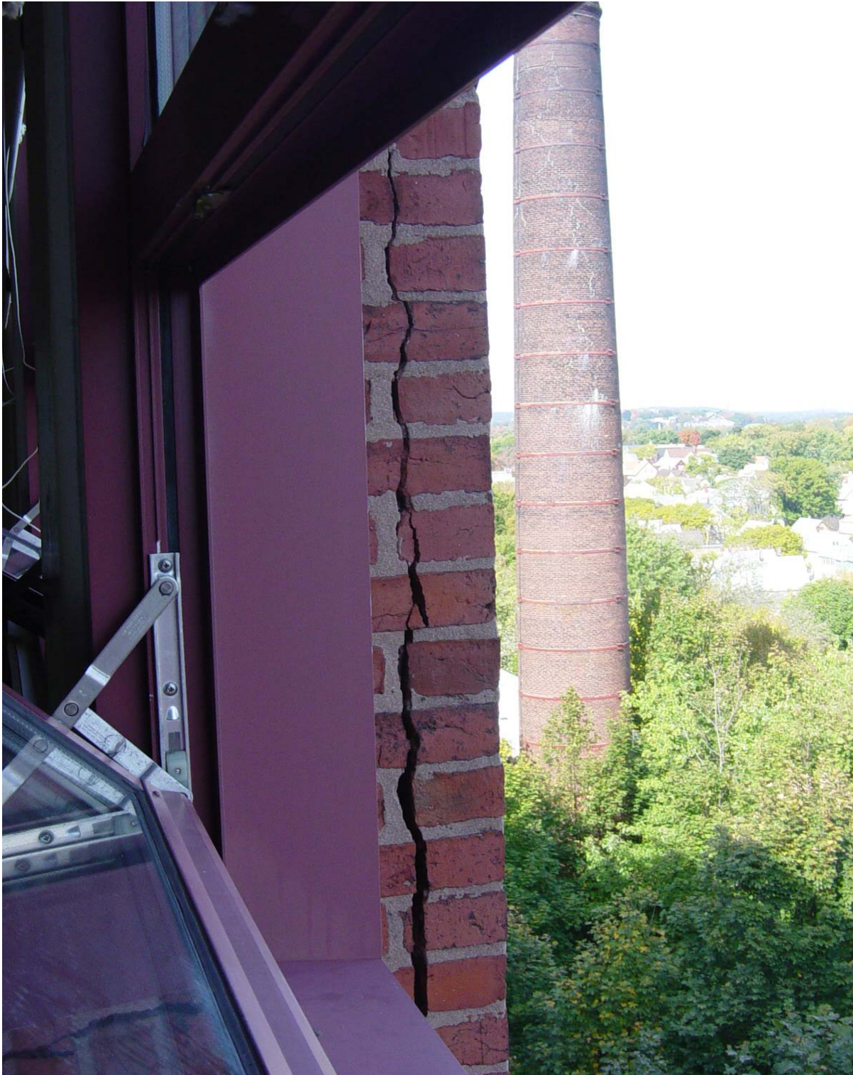
Photo 30 - Close up of cracked brick pier between windows, which occurs in a dozen or so locations. This is most likely caused by high moisture build up within the narrow pier, causing cracking in freezing weather. Face brick at pier must be removed and rebuilt. This will disturb the existing window frames and sealants.
