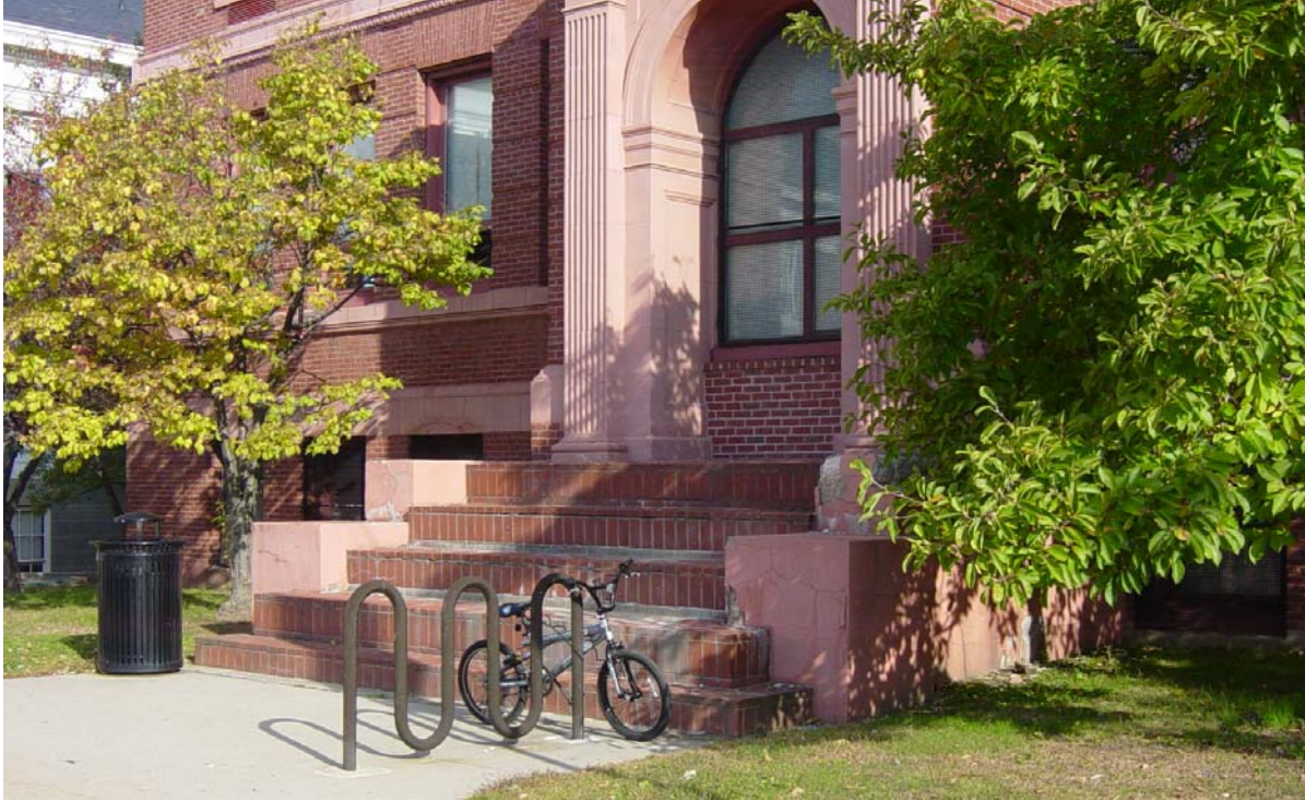
Photo 3 - Former entrance steps to west wing, converted to seating. Note deteriorated mortar and cheek walls. Entrance to east wing is similar. We recommend installing granite treads, risers and wall caps. Since the initial field investigation, the masonry steps and cheek wall have been repaired.
