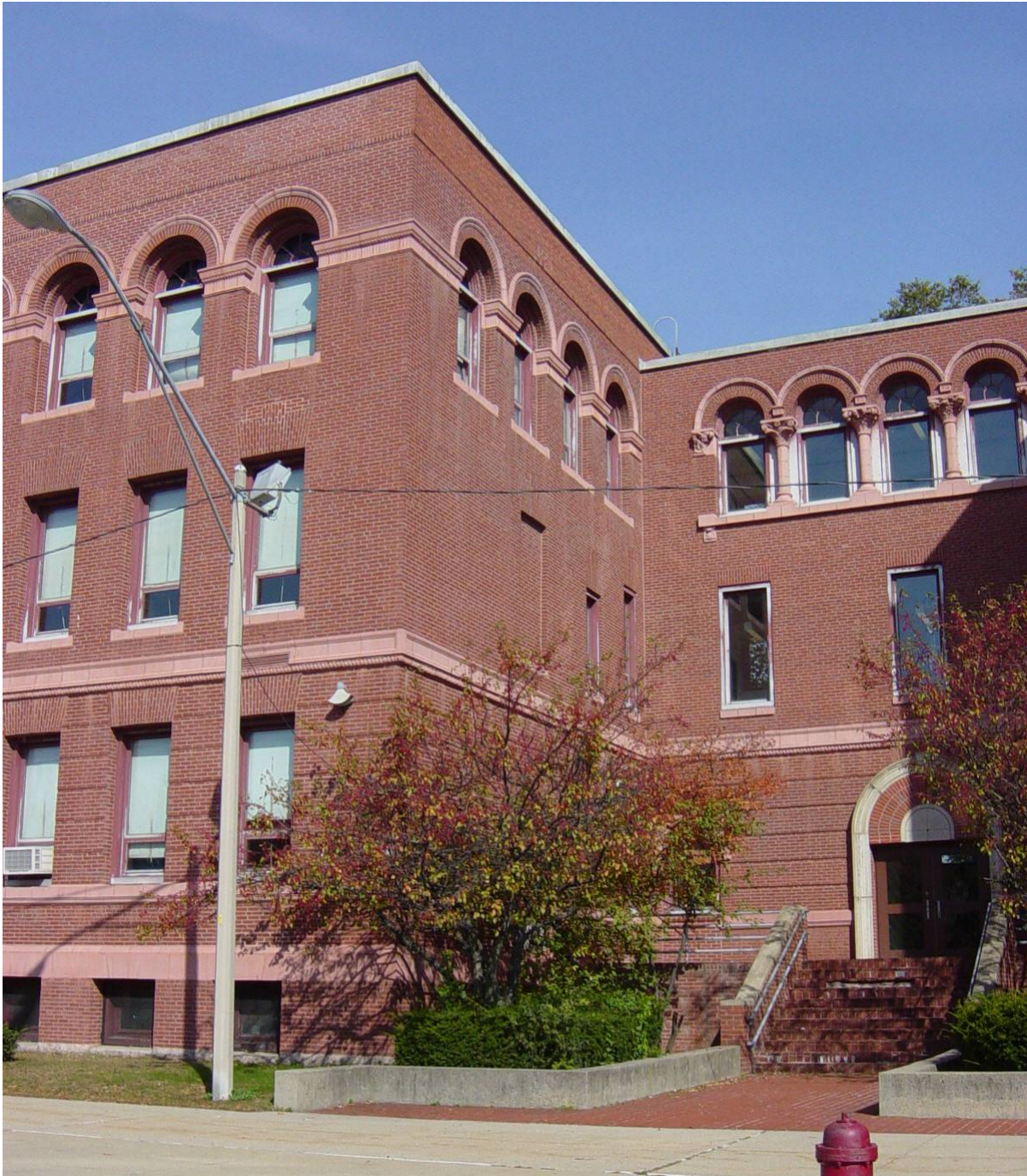
Photo 14 - Entry between east wing and original building. Wall appears in good condition. Worn finish at door, aluminum windows and panning. Arch top windows show exposed 100-year old wood frames and sashes, in poor condition. Mortar and brick failing at steps; some heaving of bricks at sidewalk
