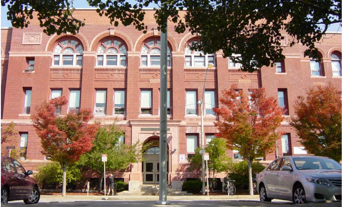
Photo 11 - Main entrance. Badly worn finish at aluminum windows and panning. Arch top windows show exposed 100-year old wood frames and sashes, in poor condition.
