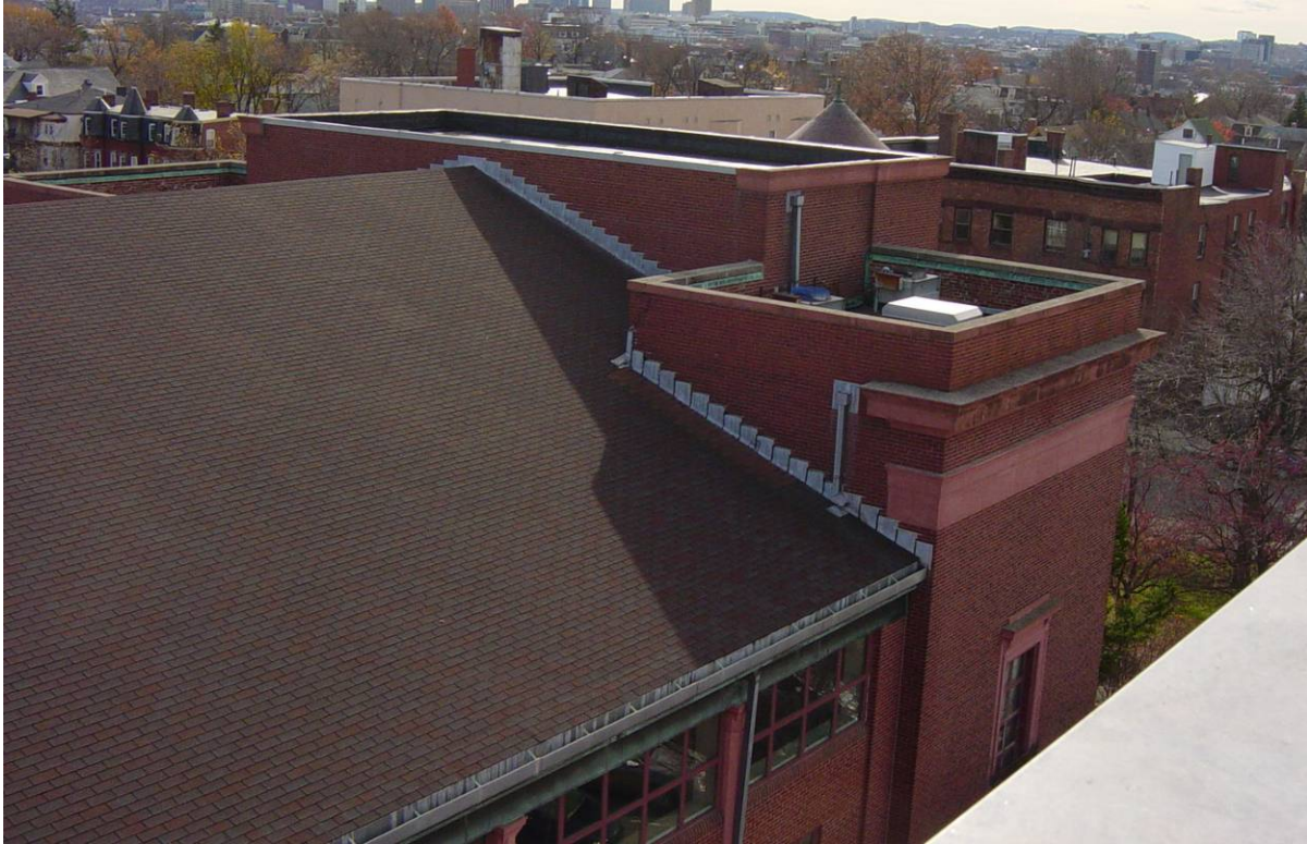
Photo 47 - Library wing. Asphalt shingle roof, gutters, flashing and flat roofs appear to be in good condition.
