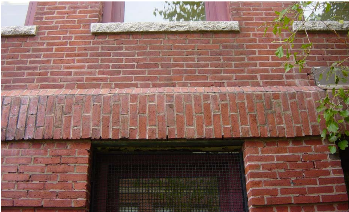
Photo 26 - Rear of building. Previous repointing job applied a thin (1/8") layer of new mortar over existing joints. Note mortar flanking the lower window, much of which is falling off. Granite sills are in very good condition. Note classroom vent on right, crudely covered over with a metal sheet.
