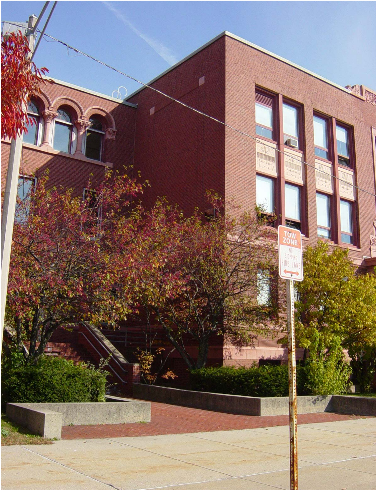
Photo 16 - Concrete site walls appears to be in good condition, but application of inexpensive clear penetrating water repellent will extend their life. Brick wall at building is in good condition.
