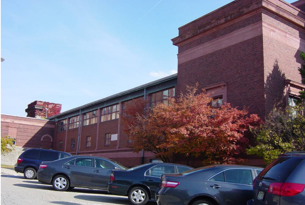
Photo 20 - West elevation of library. Windows were fully replaced in 1986, and brick walls were infilled below. Some areas of mortar and cast stone are in poor condition. Masonry cornice is badly stained.
