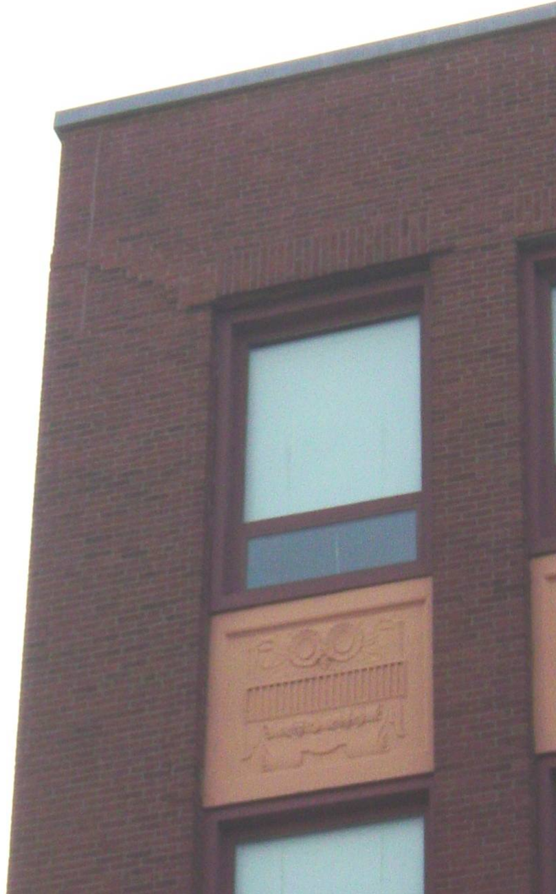
Photo 24 - Rear of building. Face brick is cracking and separating at the northeast and northwest corner of the west wing, causing the diagonal cracking seen above. Approximately 120 s.f. of brick must be rebuilt at each corner.
