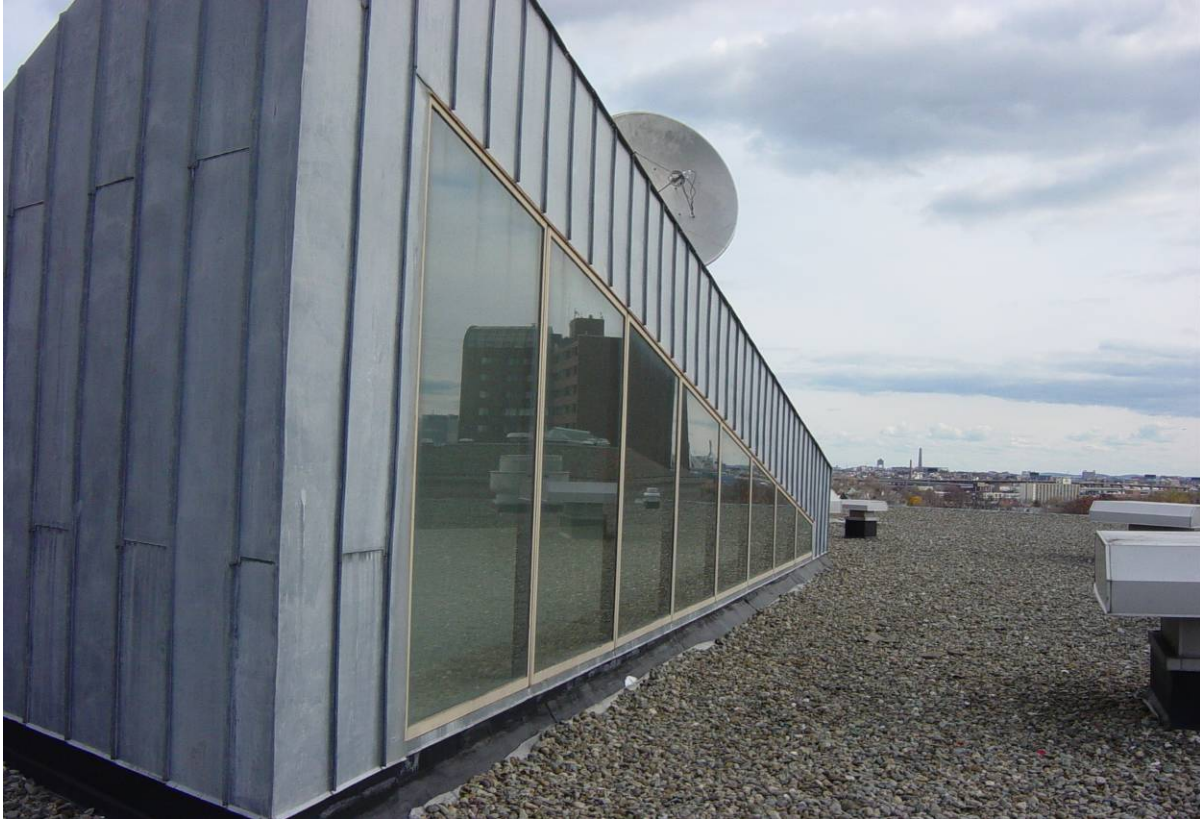
Photo 51 - Atrium monitors. EPDM curb flashing shows splits, holes and cracks. Replacement of all curb flashing is recommended.
