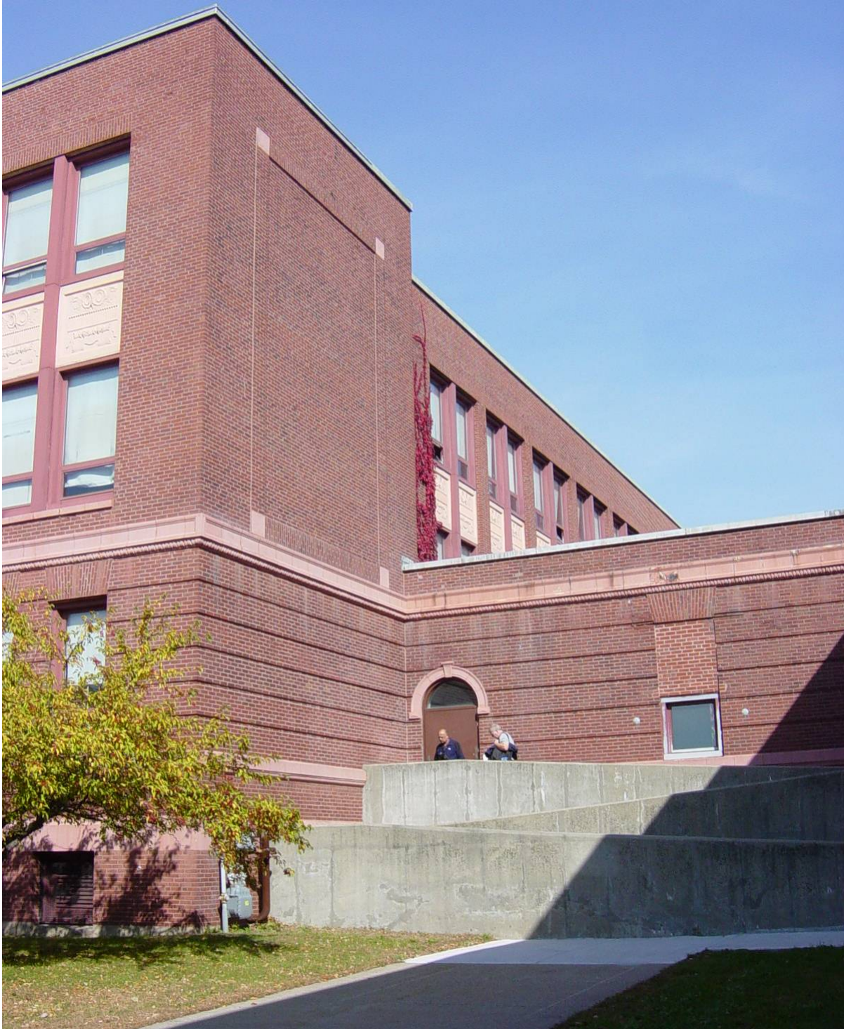
Photo 19 - East elevation of east wing, with link to library. Brick and mortar is failing at arch above square window. Concrete handicap ramp in foreground is deteriorating, appears to have been patched in many places. Applying clear penetrating water repellent to concrete is recommended.
