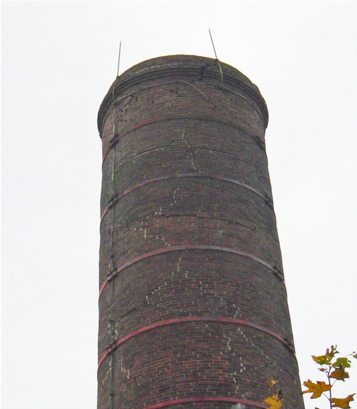
Photo 32 - Physical Plant. Smokestack shows severe cracking at top, possibly due to lightning strikes. Some cracks may be up to 8" wide. Inspection and repair is recommended. Picture taken from east side.
