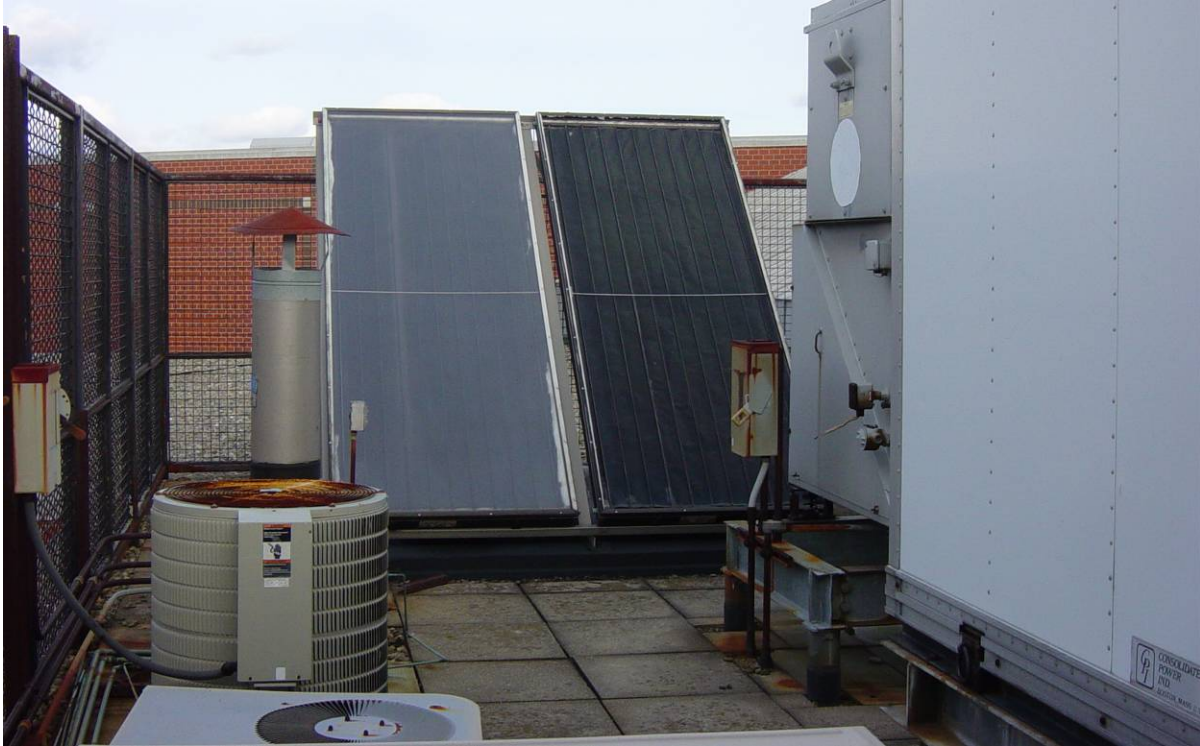
Photo 53 - Fenced in area at Technical High School Roof. Originally designed as a lab for HVAC classes, this area is cluttered with abandoned equipment. Dozens of deteriorated roof penetrations have led to water leakage into the computer lab below.
