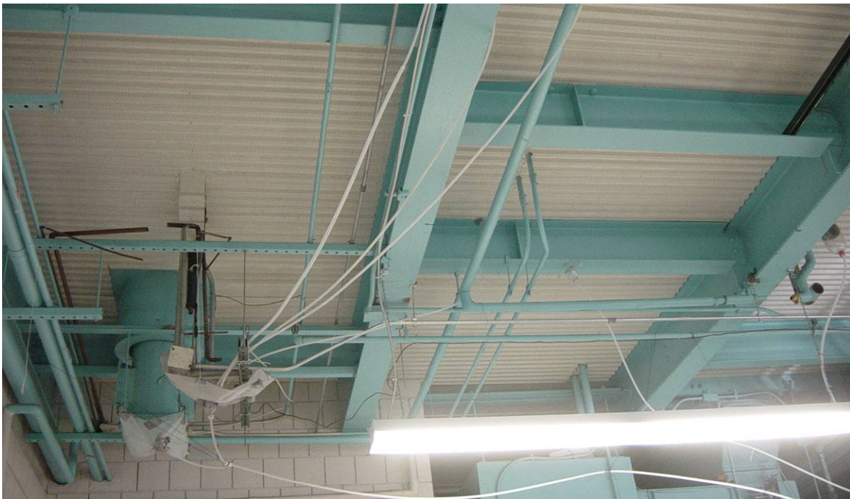
Photo 54 - Computer lab ceiling, rigged with collectors and plastic tubing to catch and direct roof leaks.
