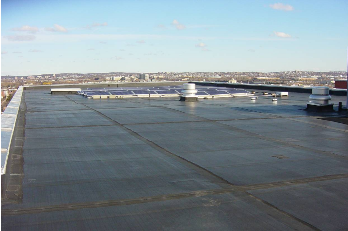
Photo 39 - West wing roof. Due to high winds and uplift forces, some areas of the EPDM membrane are experiencing adhesive failure, separating from the insulation. Many small voids were noted below the membrane. Some areas of plywood are pulling off the back of the parapets. The area of roof behind the photovoltaic cells has been recently replaced. See Sketch SK-3.
