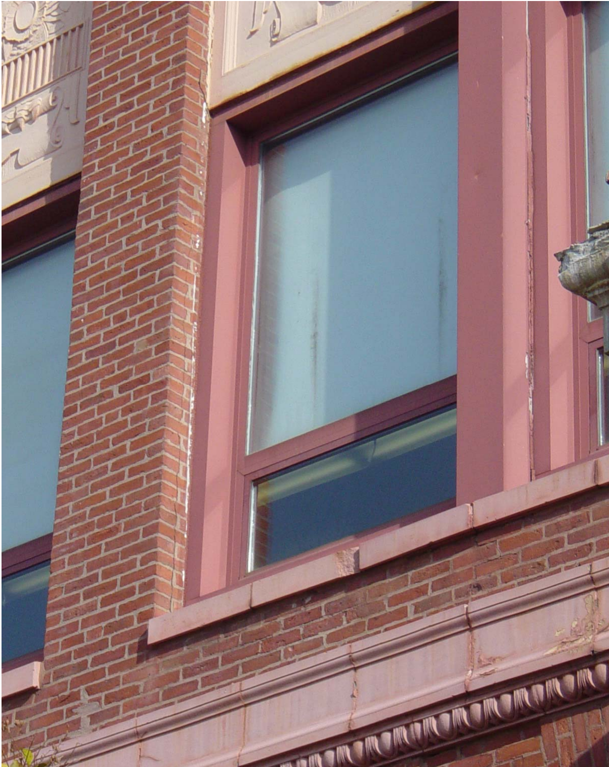
Photo 5 - Vertical cracking of brick pilasters between windows is a common problem, as is cracking at window sills, sealant failure at window panning, and rusting at lintels. At far right, masonry cornice is badly deteriorated. All are in need of repair.
