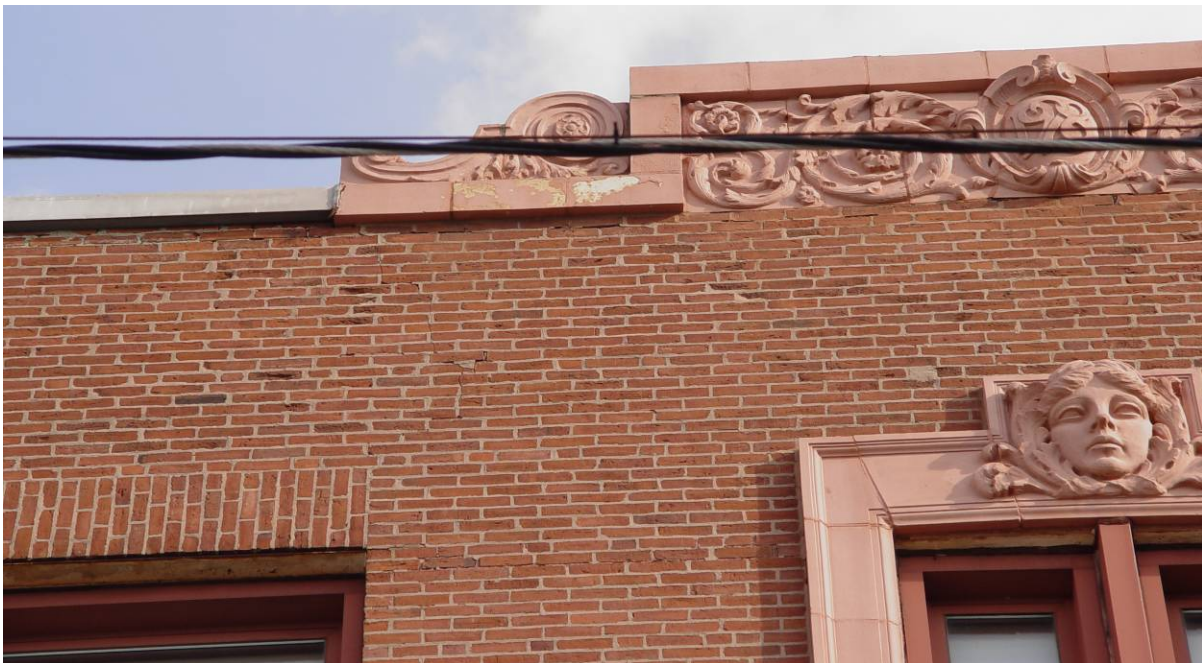
Photo 4 - Close-up shows extensive cracking of brick and mortar. Coating is peeling at masonry details; lintels are rusting. All are in need of repair.
