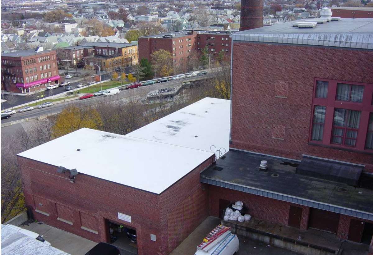
Photo 43 - Physical Plant. New PVC roof installed summer 2010. Roof over receiving is from 1986.
