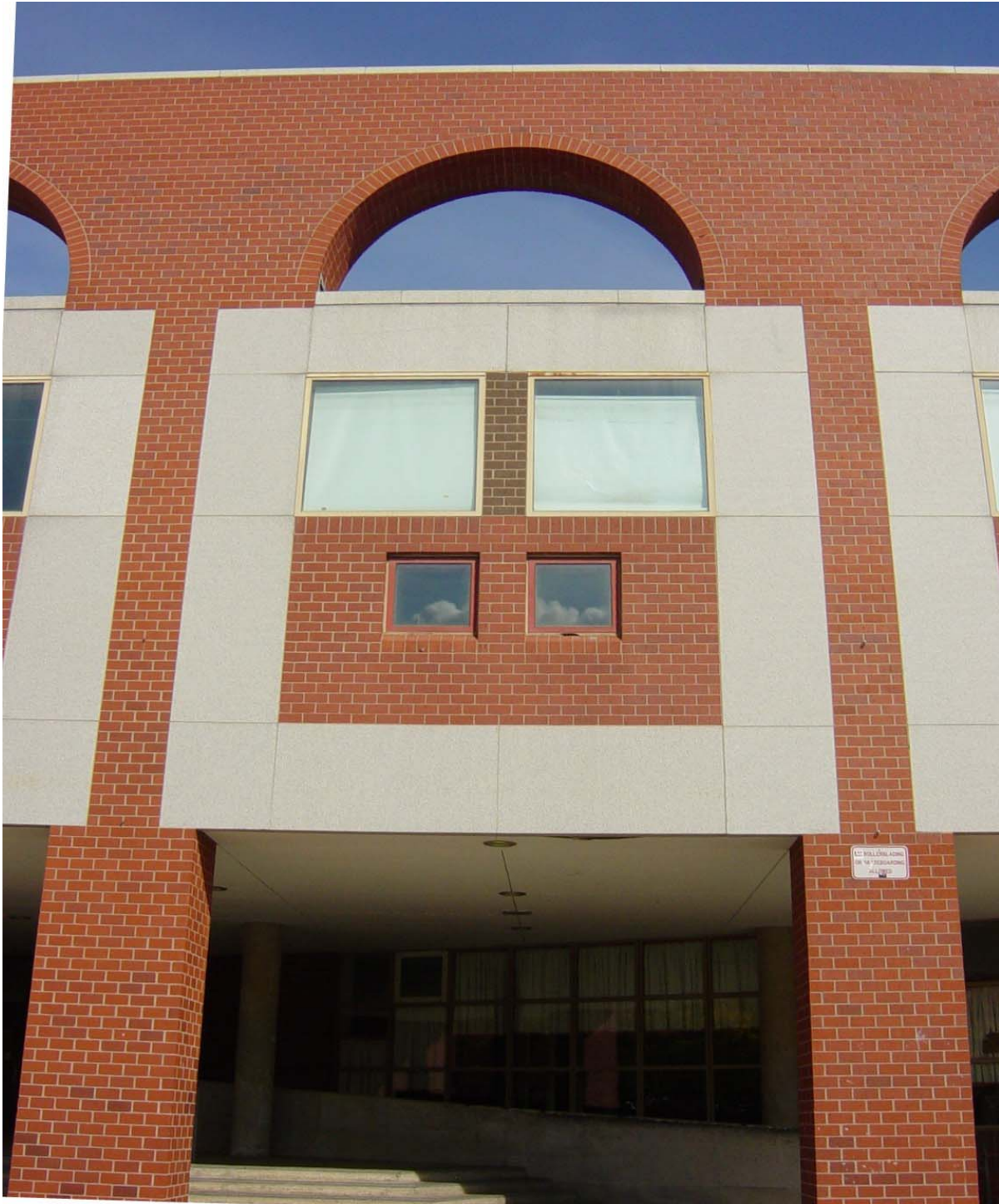
Photo 34 - Technical High School entrance. The exterior masonry walls are in very good condition and require only minor work. Some areas of stucco soffit are failing and need repair.
