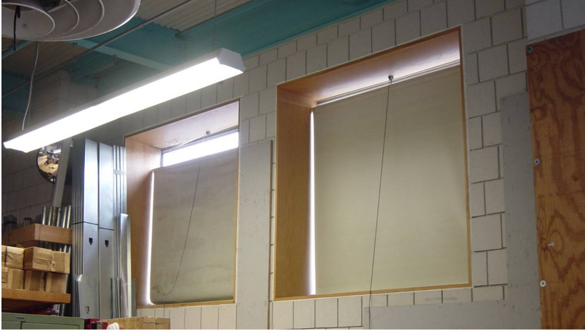
Photo 37 - Electrical Shop. Some windows show severe deterioration at the heads due to moisture; others do not. Indicates improperly detailed and installed head flashing.
