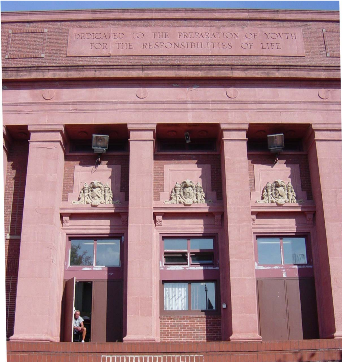
Photo 22 - Library entrance. Cast stone has been coated with light terra cotta colored treatment, likely applied in 1986. Large amounts of spalling of the cast stone is visible behind the treatment, evidence that moisture is getting trapped.
