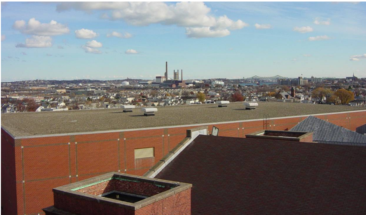
Photo 48 - Foreground: Library wing. Deterioration seen at copings, joints and flashings. Roof hatch left open. Background: Ballasted roof at Technical High School gymnasium.
