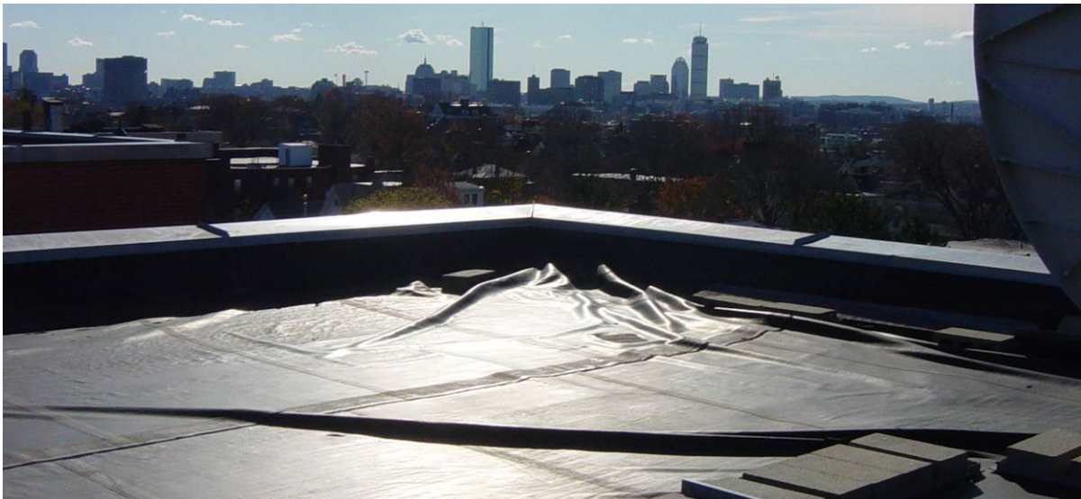
Photo 40 - West wing roof. Due to high winds and uplift forces, some areas of the EPDM membrane are experiencing adhesive failure.
