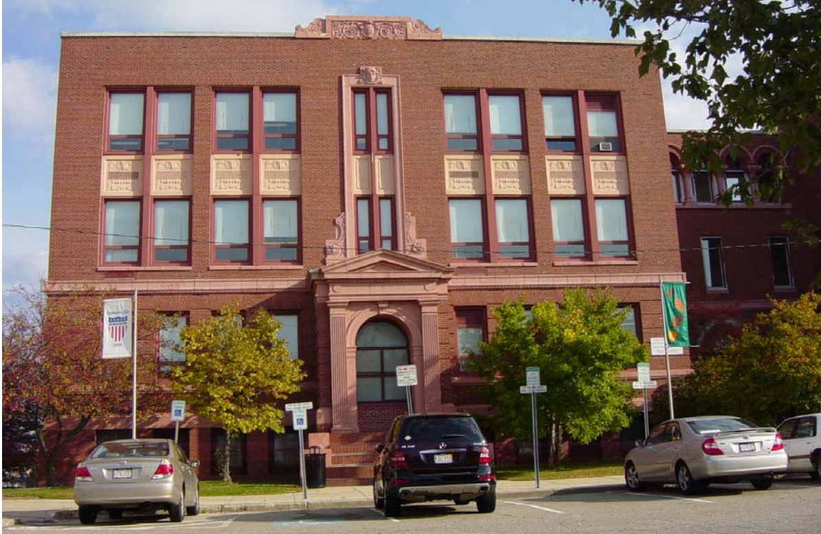
Photo 1 - South elevation of west wing. Terracotta spandrels are in good condition.
