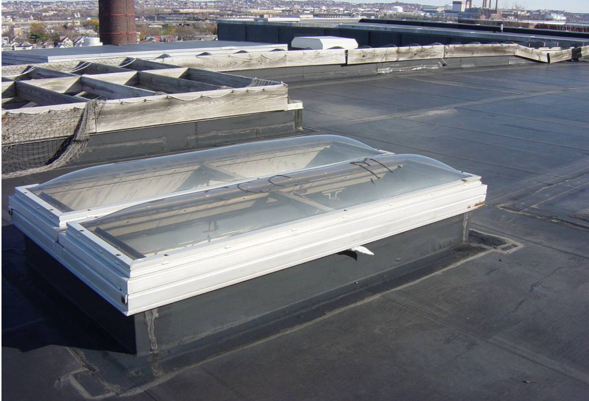
Photo 45 - Central wing, north. Curb flashing is severely deteriorated in locations such as roof hatches and the bird netting support structure. Several patches are seen. Netting and support structure are damaged in some areas. Roof at auditorium beyond appears to be in very good condition.
