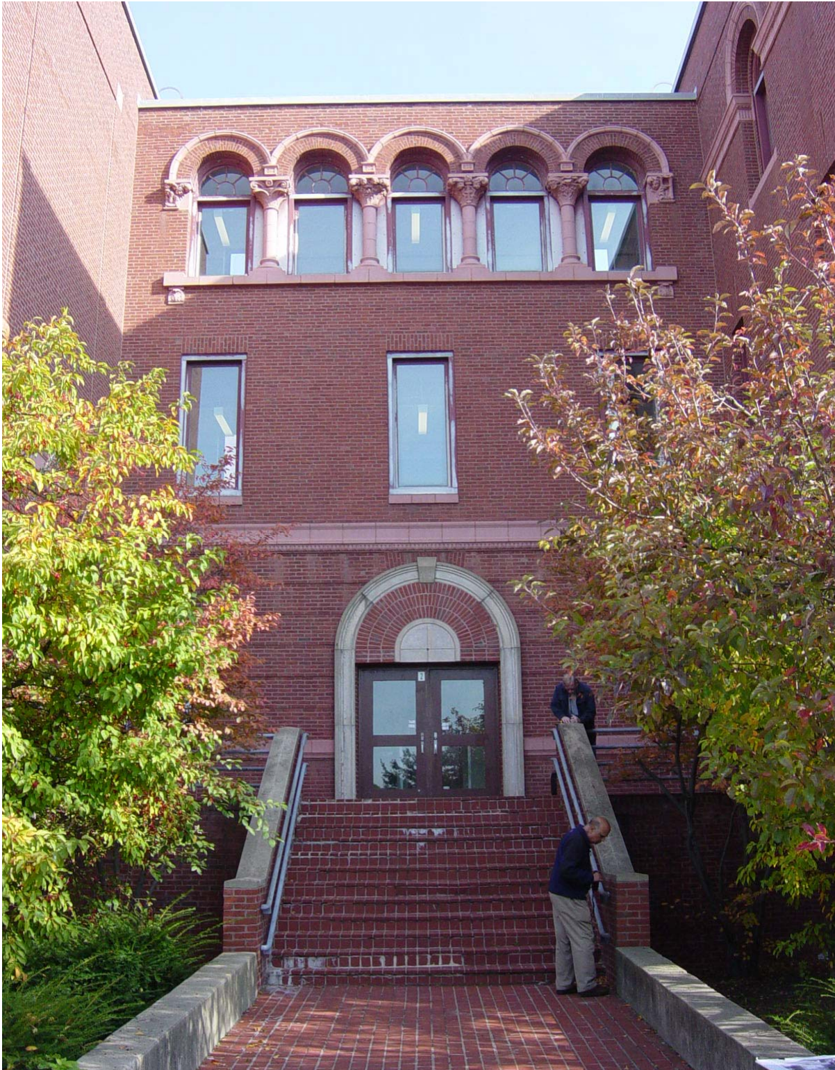
Photo 7 - Entry between west wing and original building. Walls are in good condition. Worn finishes at door, window frames and panning. Arch top windows show exposed 100-year old wood frames and sashes, in poor condition. Mortar and brick are failing at steps; some heaving of bricks at sidewalk. Since the initial field investigation, the masonry steps and cheek wall have been repaired.
