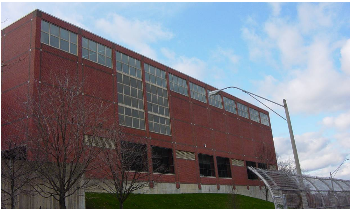
Photo 36 - Rear of Technical High School Gymnasium. Northern exposure makes wall and windows vulnerable to wind driven rain. Reports of water leakage on the inside of this wall during rains.
