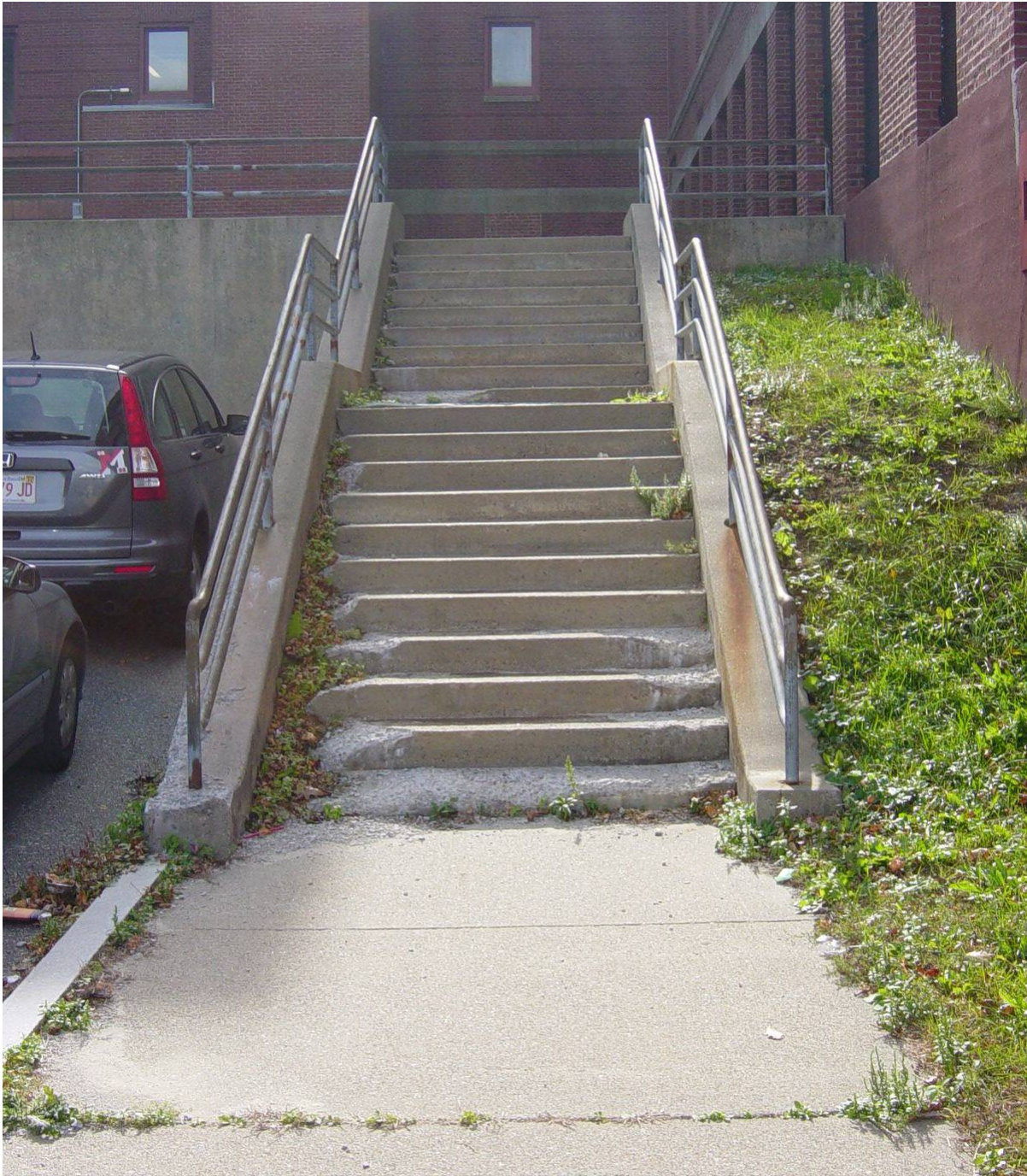
Photo 31 - Rear of building. Stair has deteriorated badly and is hazardous to walk on. Cheek wall/retaining wall is sound, with superficial deterioration. Railings are rusting. Reconstruction of stairs, repair of wall and refinishing of railings is recommended.
