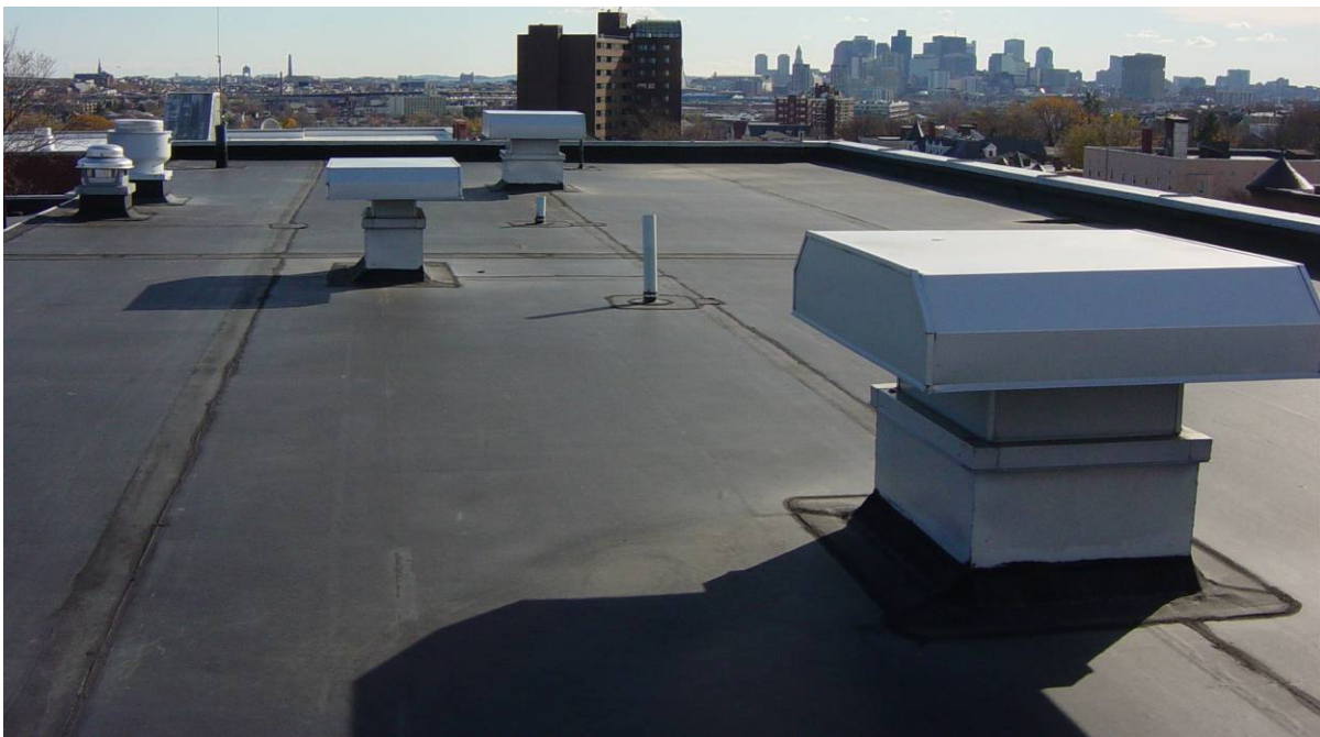
Photo 44 - Central wing, south. Existing roof is well adhered and in good condition.
