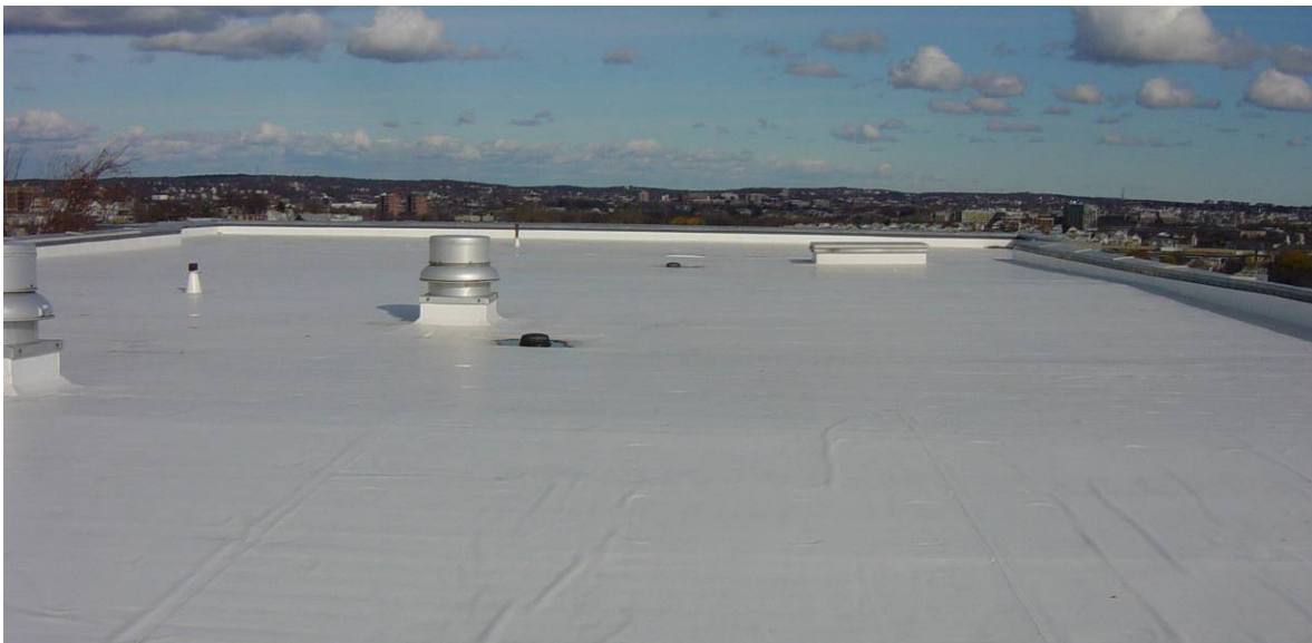
Photo 46 - East wing. New PVC roof with RhinoBond fasteners installed summer 2010.
